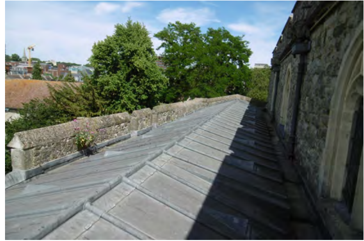
THE NORTH AISLE (CHANCEL) ROOF
