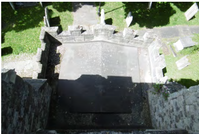
THE NORTH PORCH ROOF
