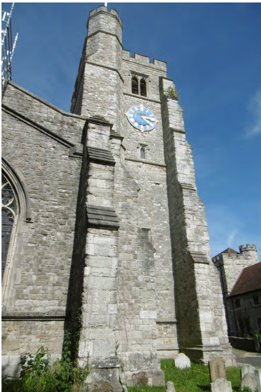
THE WEST ELEVATION OF THE TOWER
