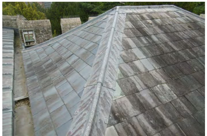
THE VESTRY ROOF
