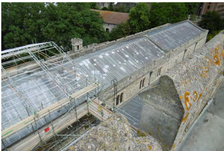
THE NAVE AND CHANCEL ROOF
