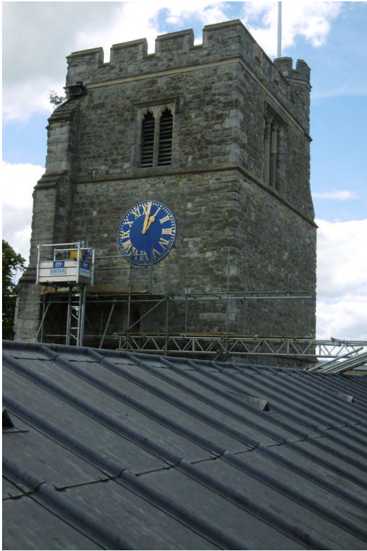
THE EAST FACE OF THE TOWER
