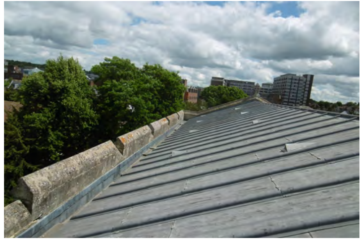
THE CHANCEL ROOF
