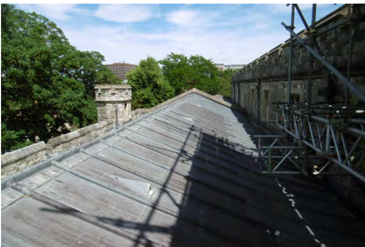
THE NORTH AISLE (NAVE) ROOF
