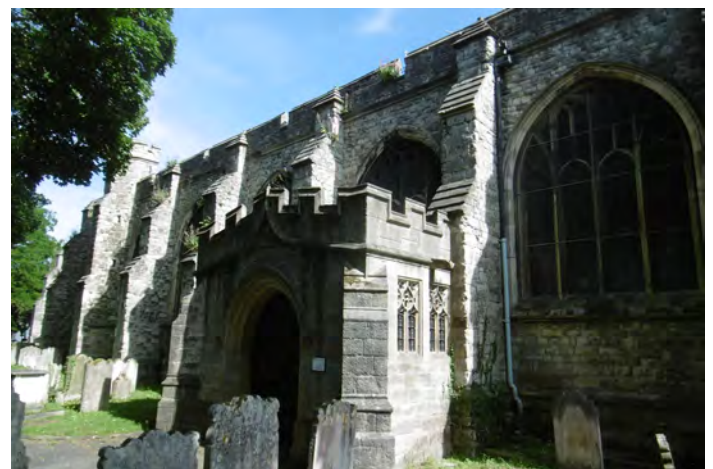
THE NORTH AISLE
