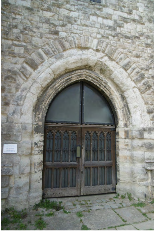
THE SOUTHTOWER DOOR
