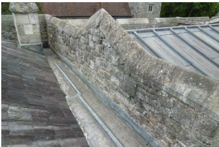
THE ORGAN LOFT PARAPET
