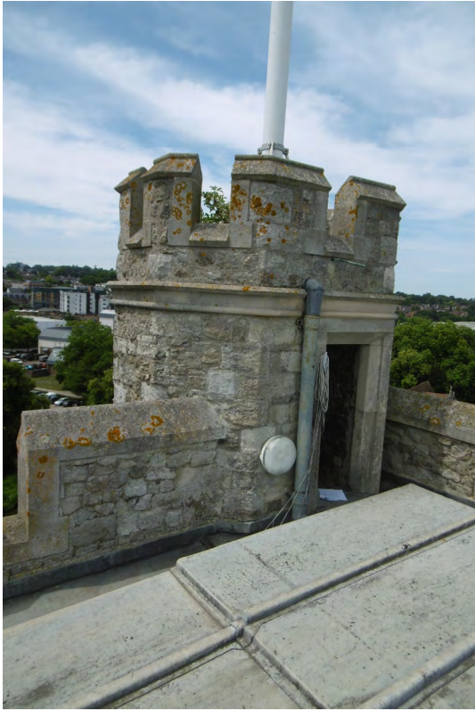
THE TOWER ACCESS TURRET
