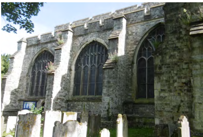
THE NORTH ELEVATION OF THE NORTH CHANCEL AISLE
