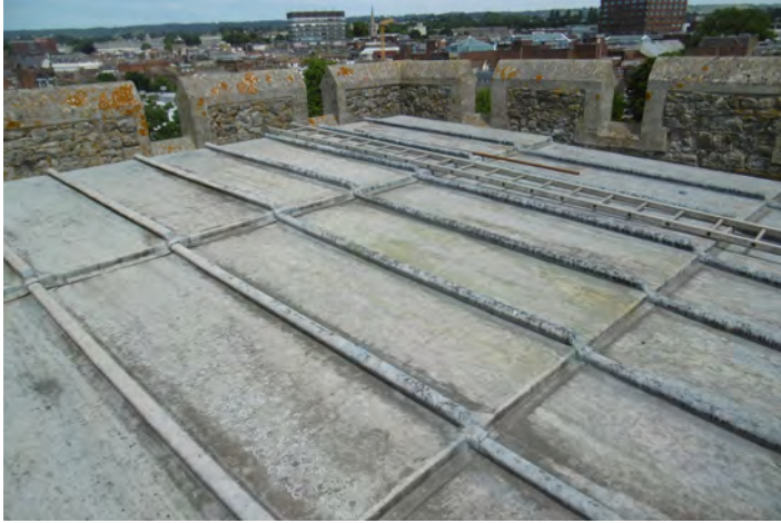
THE TOWER ROOF
