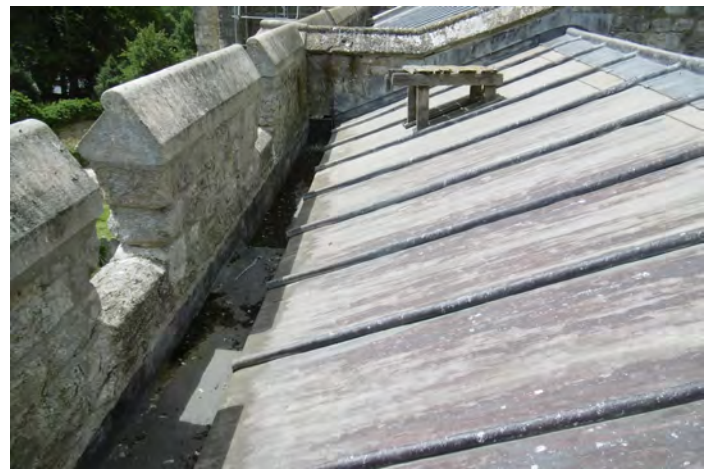
THE ORGAN LOFT ROOF
