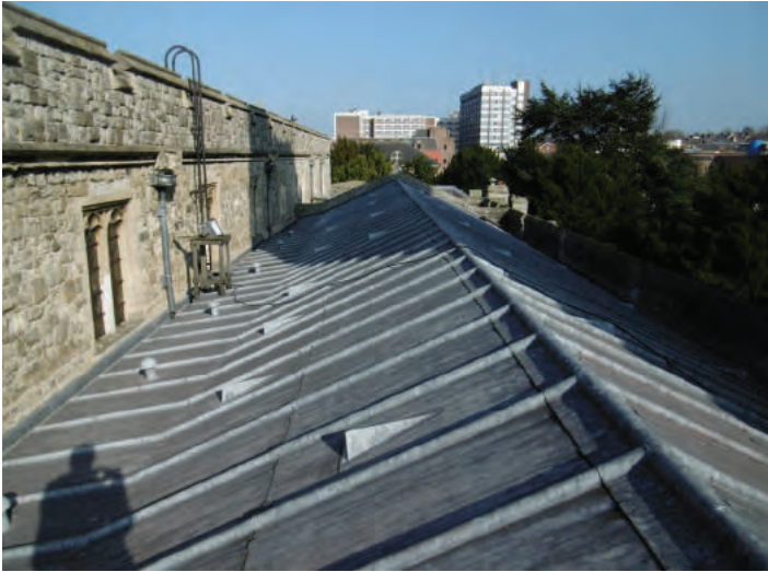
THE SOUTH AISLE ROOF
