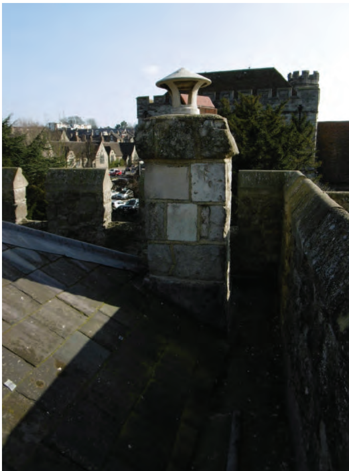
THE BOILER HOUSE CHIMNEY
