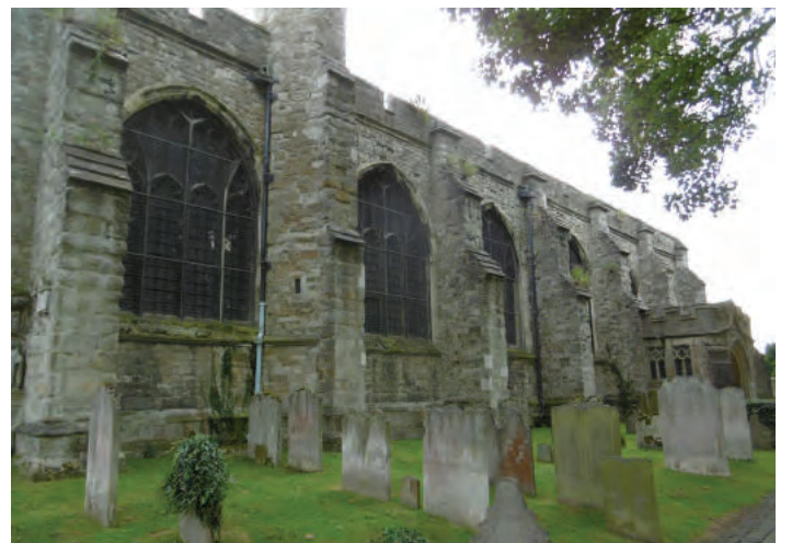
THE NORTH ELEVATION NORTH AISLE
