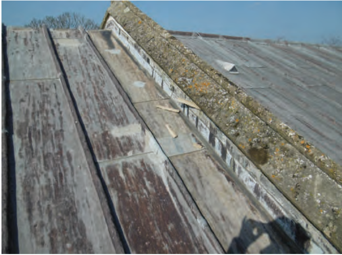
THE NAVEL ROOF GABLE PARAPET
