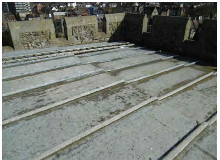
THE TOWER ROOF
