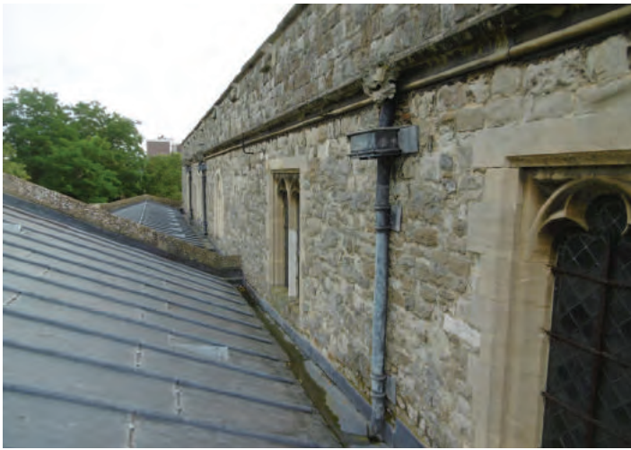
THE NORTH CLERESTORY
