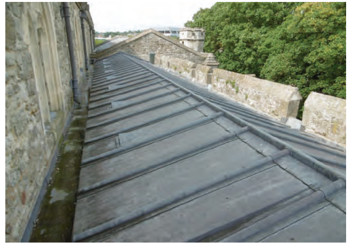
THE NORTH CHANCEL AISLE
