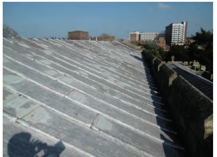
THE NAVE ROOF
