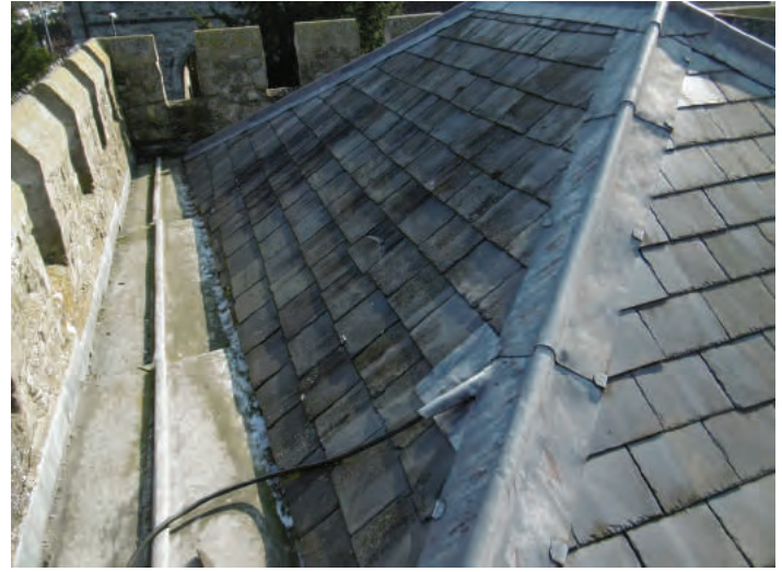
THE VESTRY ROOF
