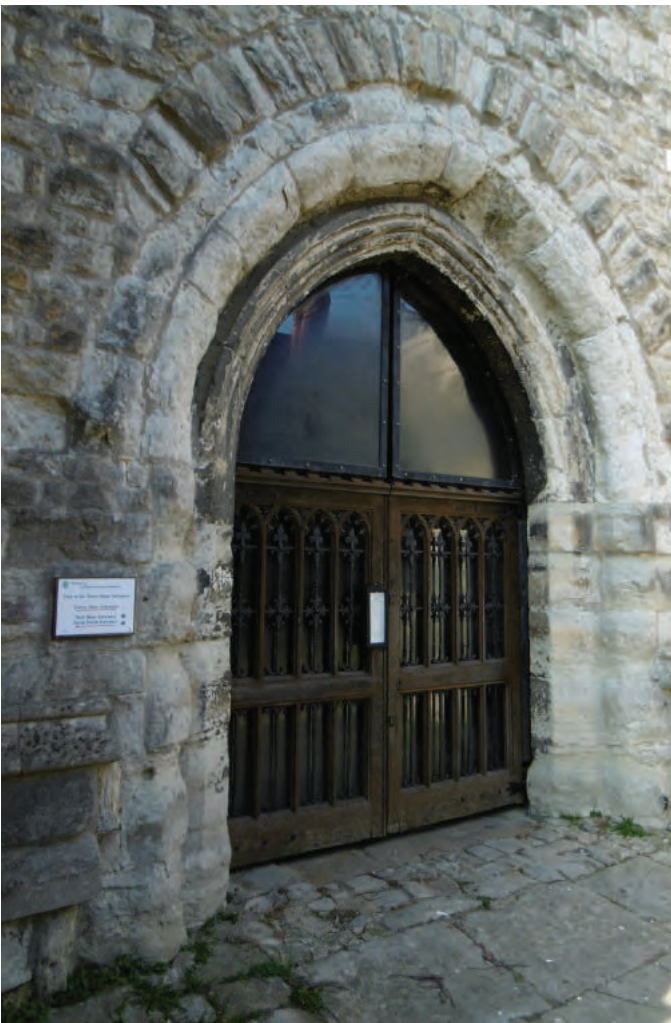
THE TOWER DOOR
