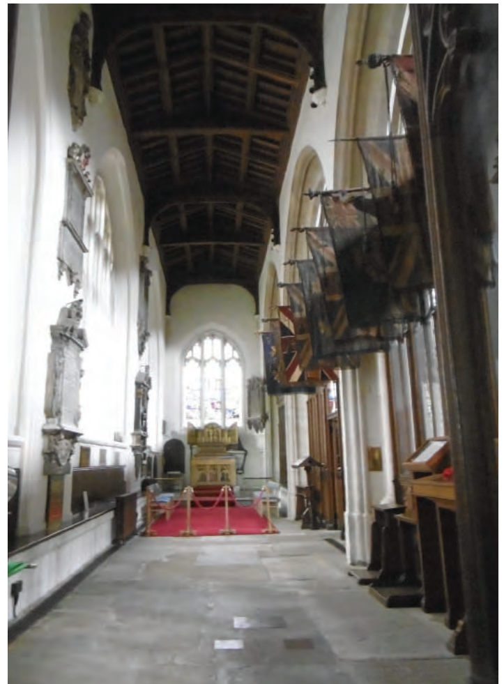
THE NORTH CHANCEL AISLE
