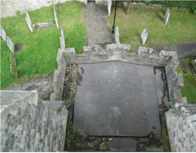
THE NORTH PORCH ROOF
