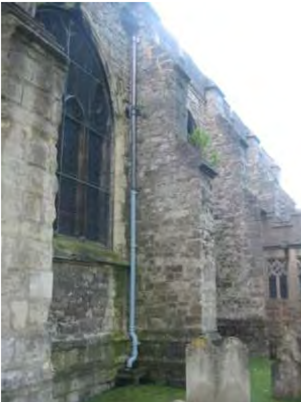
Stone work to the Nave North Aisle
